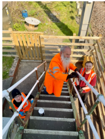
The CRP team, Brian, Catherine and Max refurbishing the external staircase.
